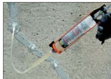
Crack-Pac® Injection using the E-Z-Click Port System
